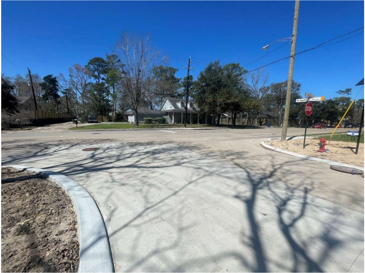
Figure 7.2 Burkhardt Rd Intersection
