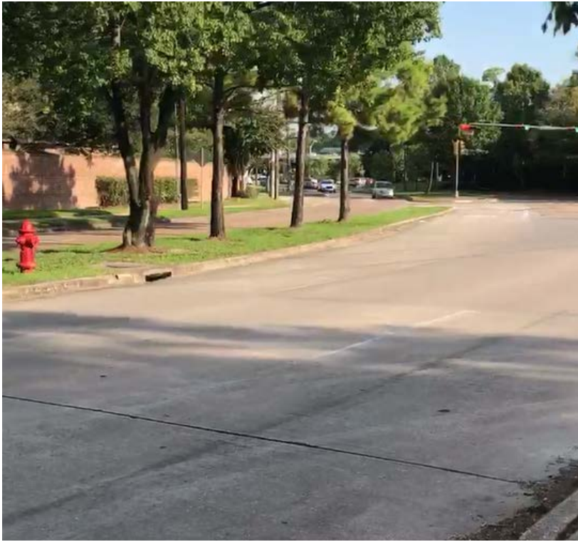
Figure 1: Driveway sight line looking south.
