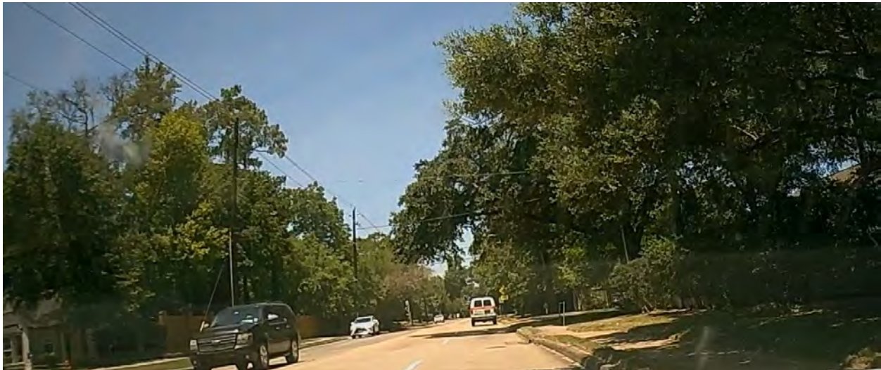
Figure 1 – Driver View of the Ped Crossing from 260' South of the Crossing, Traveling Northbound – The control devices and pavement markings at the crossing can barely be seen. The required stopping sight distance is 305 feet upstream of the crossing where drivers are supposed to clearly see the control devices and waiting area of pedestrians.
