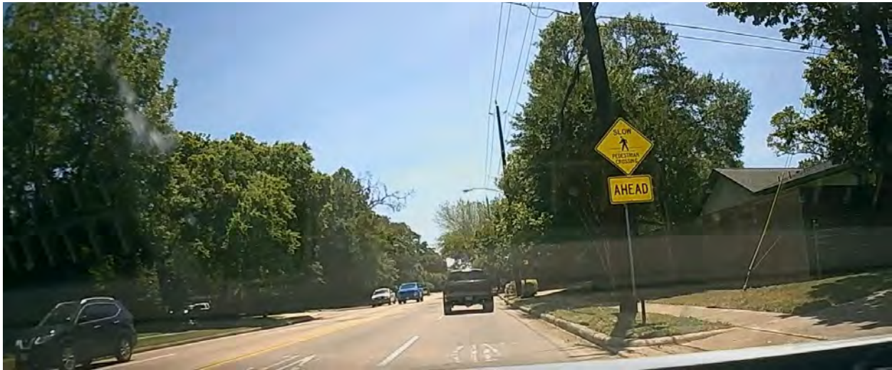
Figure 2 – Driver View of the Ped Crossing from 110' North of the Crossing, Traveling Southbound – The control devices and pavement markings at the crossing can barely be seen. The required stopping sight distance is 305 feet upstream of the crossing where drivers are supposed to clearly see the control devices and waiting area of pedestrians.
