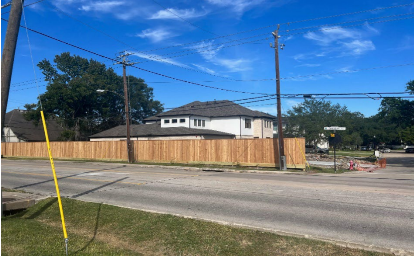
9022 Lupton Court – 8 foot wooden fence running bordering Campbell running along side yard and into front yard property line.
