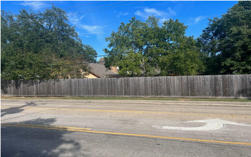
9023 Lupton Court – 7 foot wooden fence bordering Campbell running across backyard property line.
