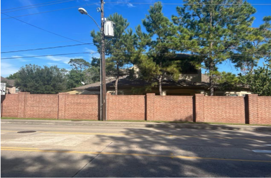
5 Cardwell Court – 8 foot brick fence bordering Campbell on side yard property line.
